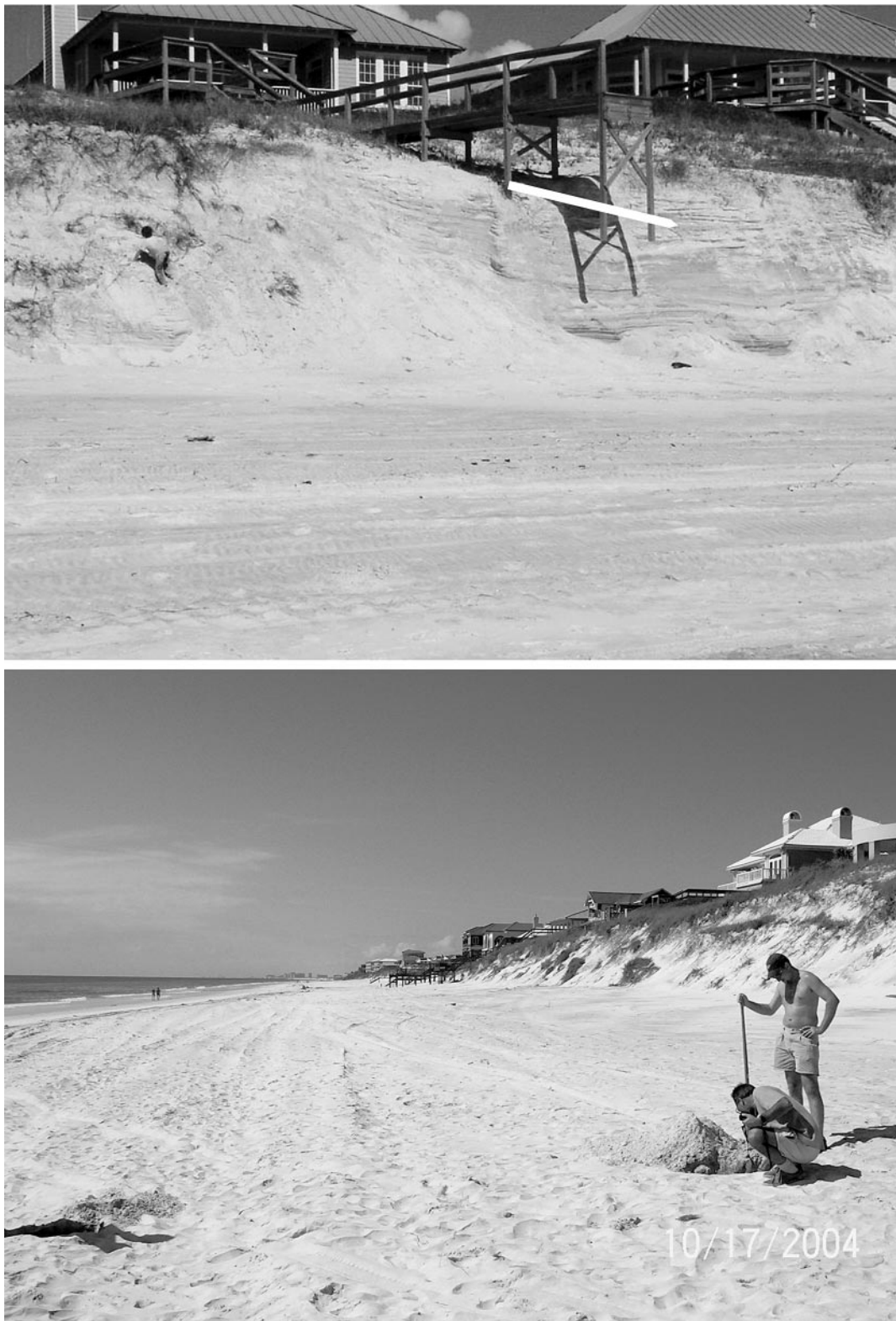
Figure 3. Study site S2-GVH. Upper: dune scarp with white line indicates prestorm dune level at the walkover structure (distinguished by the different color of the wood); lower: extensive dune scarp and locations of the trenches. Photo was taken on October 17, 2004, 30 d poststorm.
